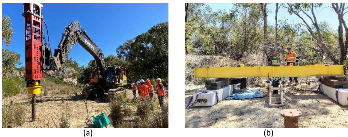
Figure 4 Pile testing in cemented carbonates: (a) pile driving, (b) tensile loading
