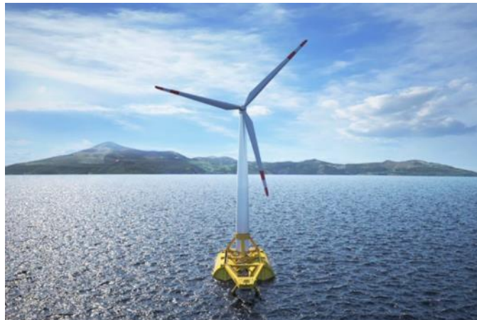
Figure 1 Saitec Offshores SATH (Swinging Around Twin Hull) technology 2 MW turbine deployed at the Biscay Marine Energy Platform (BIMEP) off Bilbao, Spain [2].
