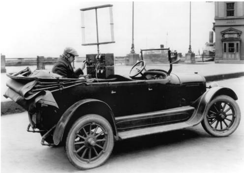
Figure 2-10 The first version of a mobile radio telephone (1924) (Lucent Technologies 2002 WWW site)
